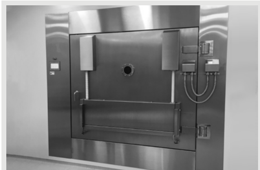
Sub door(Pizza door) system
